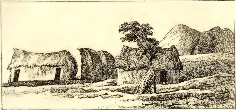
MEETING HOUSE & M r ALBRICHT'S HOUSE, FELLA.
